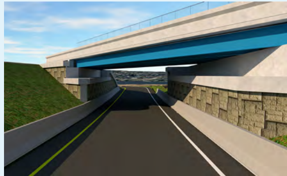
Figure 4-13: MSE Wall Visualization
